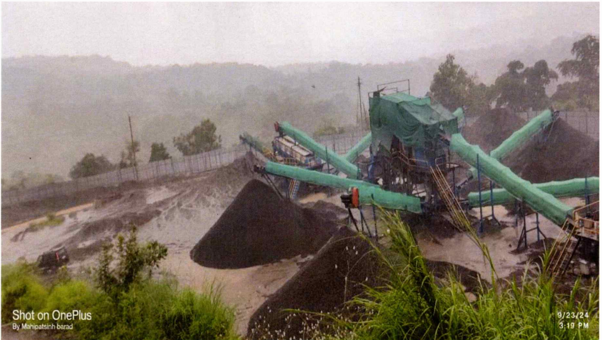
Photograph showing existing plant are covered by Green Net sheet.
